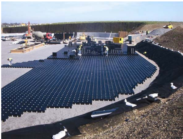
Figure 1. Constructing the geo-cellular runoff storage cell.
